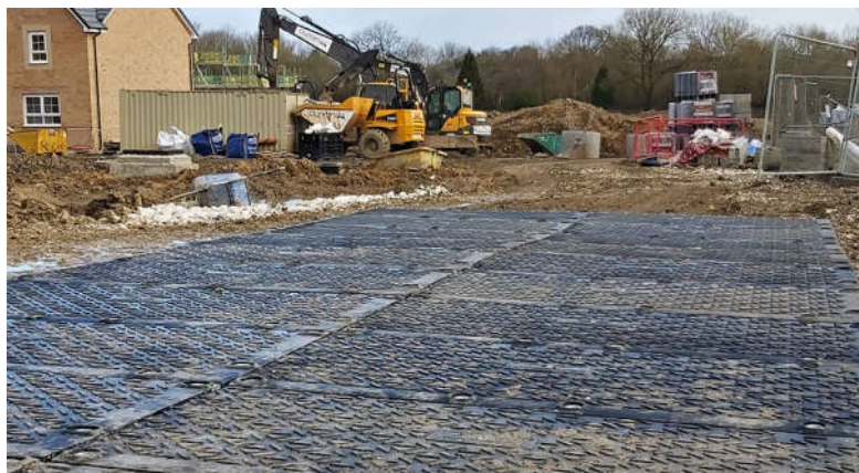
Figure 2: Ground protection mats (© GroundGuards https://www.ground-guards.co.uk/product/maxitrack-1-8m-x-0-9m-6x3/ )
